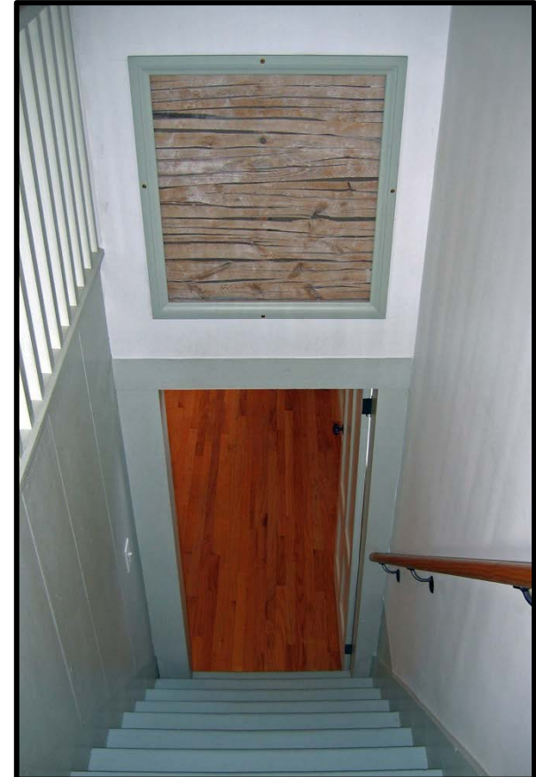
Descending from the Gallery, the split lathes were framed to show the original construction
